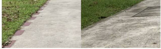
Figure 6. Closeup images of a typical shared path (left) and pedestrian path. Note the similarities, with the distinguishing feature being dotted red markings along the edges of the shared path.
